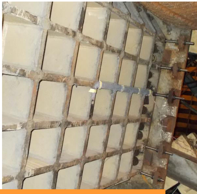
GRPF pressure Chute
